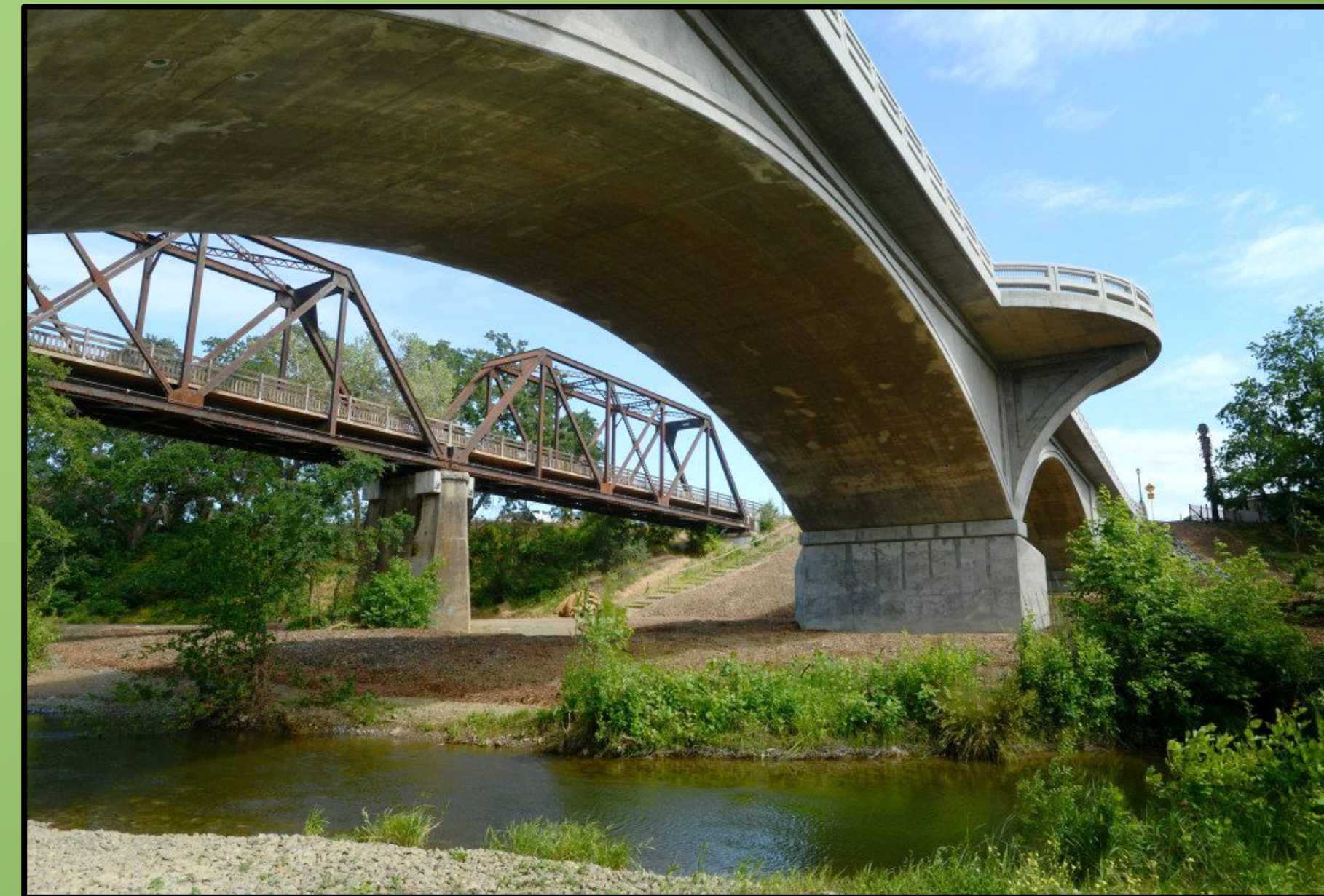
Image: Railroad Bridge (rear) and newly built Putah Creek Bridge (front) located in Winters, CA
